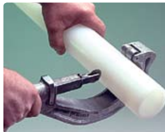
Figure 2: Cut the Tubing
