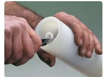
Figure 3: Chamfer the Tubing
