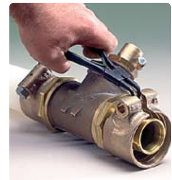
Figure 4: Dismount the Outer Sleeve
